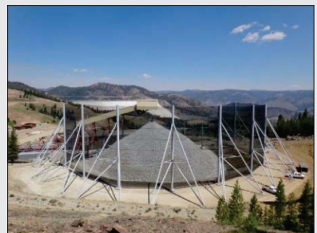
Wind Fencing around ore pile
