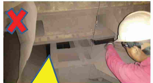
Openings below the Screen
